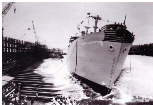
Figure 3. Sideways launching of 'William Crompton' at New Orleans.
