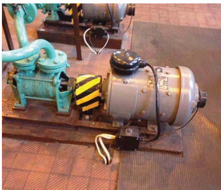
Figure 3. Outboard water pump.
